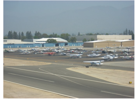
Aircraft parked on the new tie down ramp just completed at WHP
